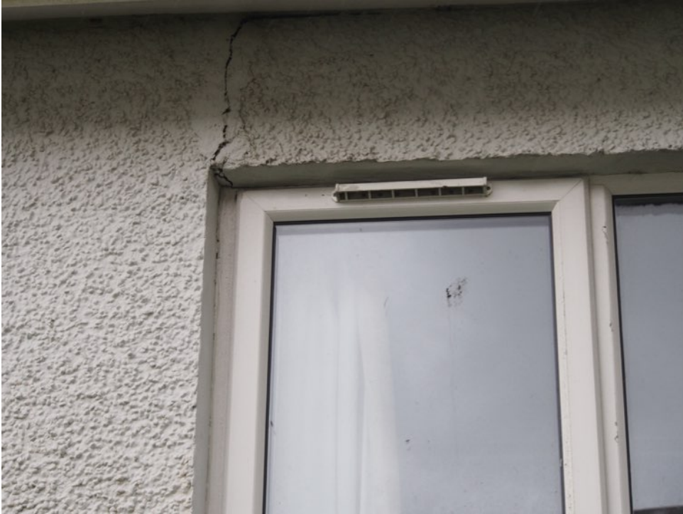
Typical crack above window, north elevation
