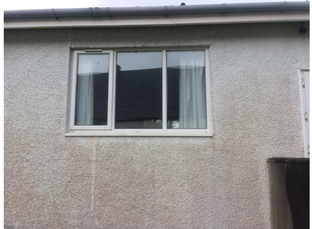
Partial north elevation showing cracks
