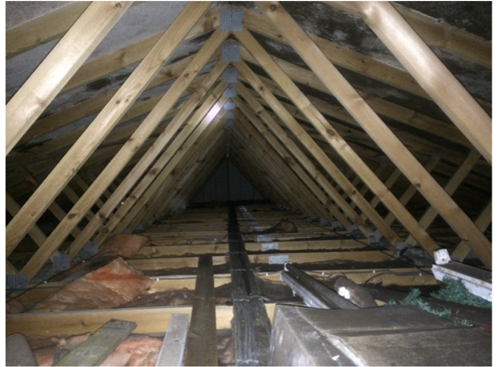
Roof space showing all sarking damp
