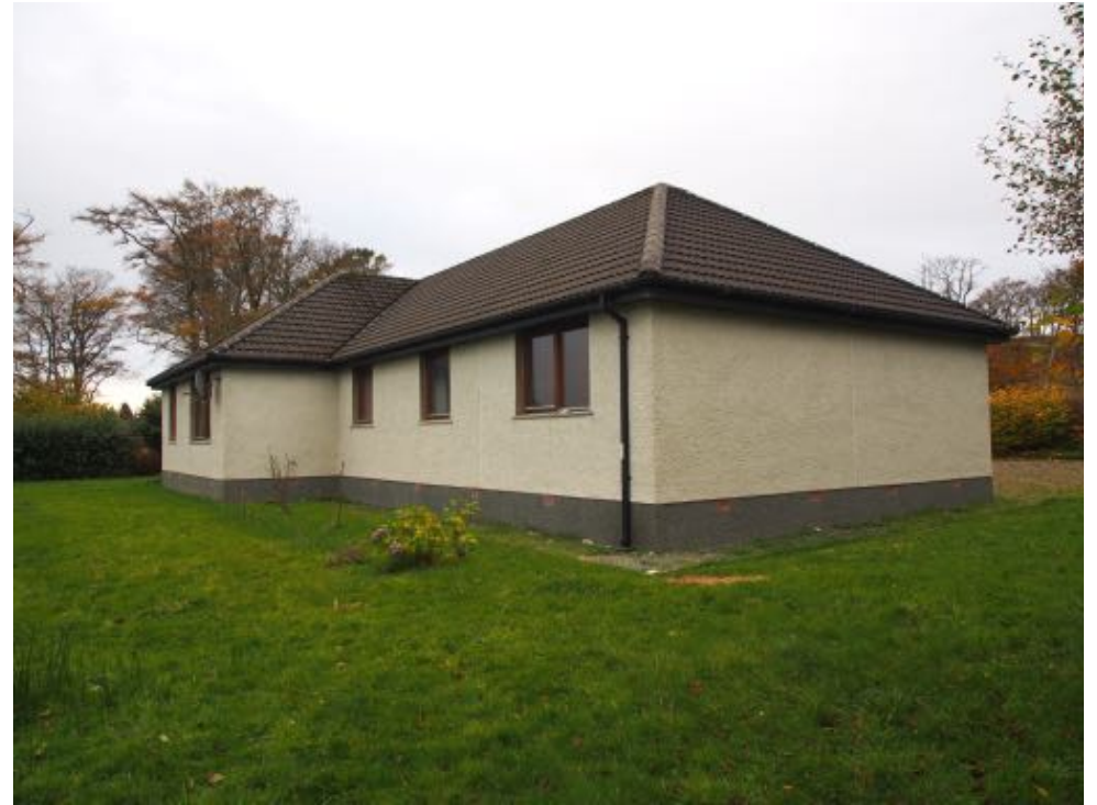
View from North
