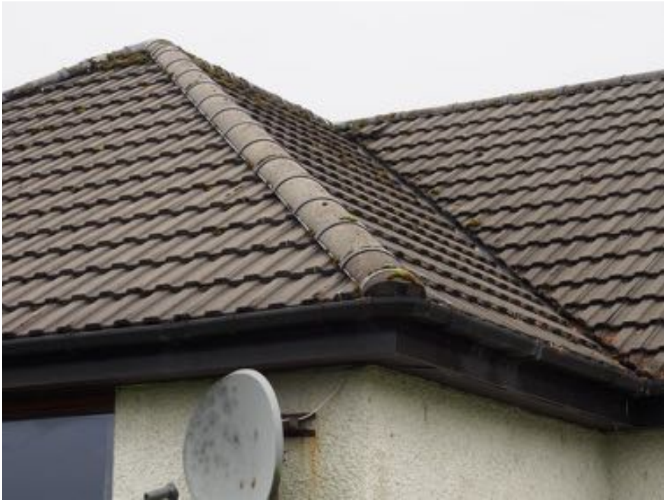
Roof tiles on South East elevation
