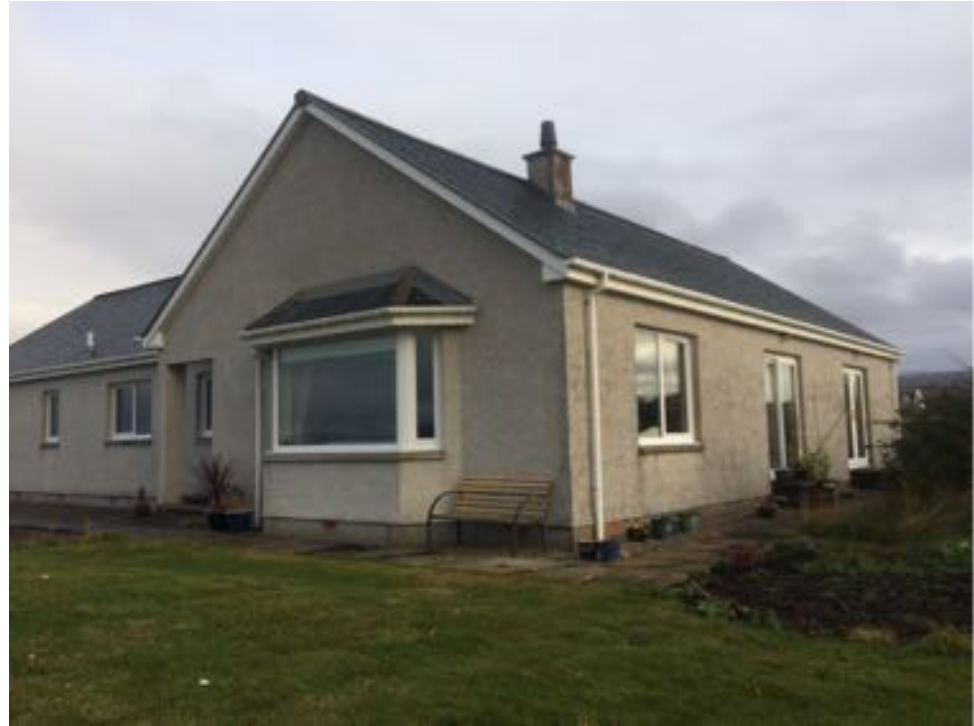
North West corner
