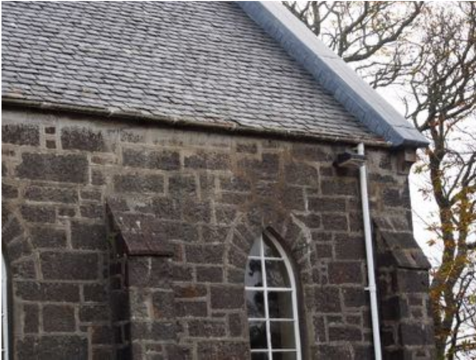
West elevation buttresses and window head
