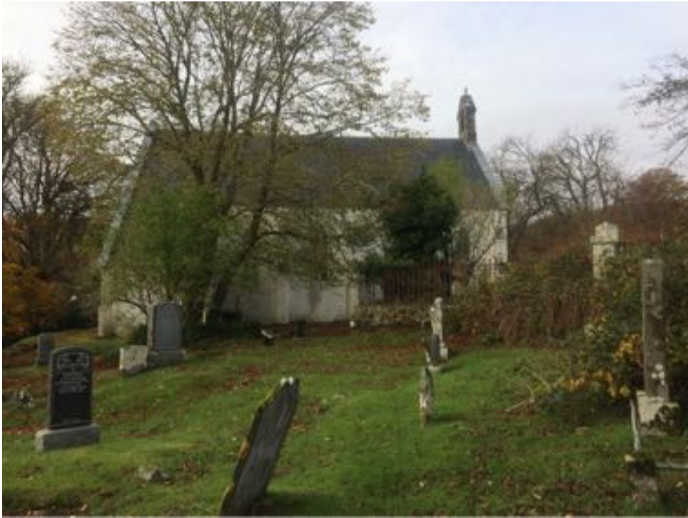
View from church yard on East side
