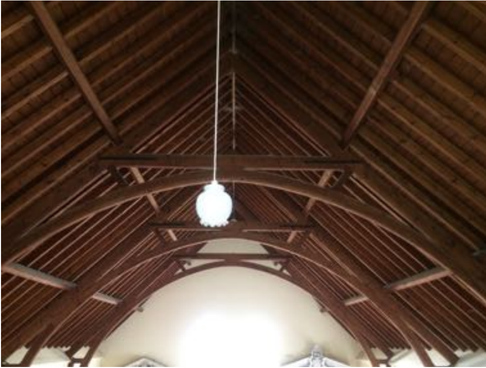
Roof structure, view looking South
