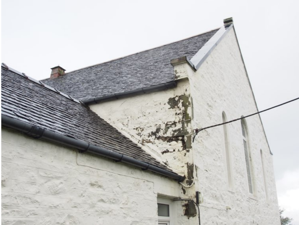
Damaged paint finish at South East corner of main church
