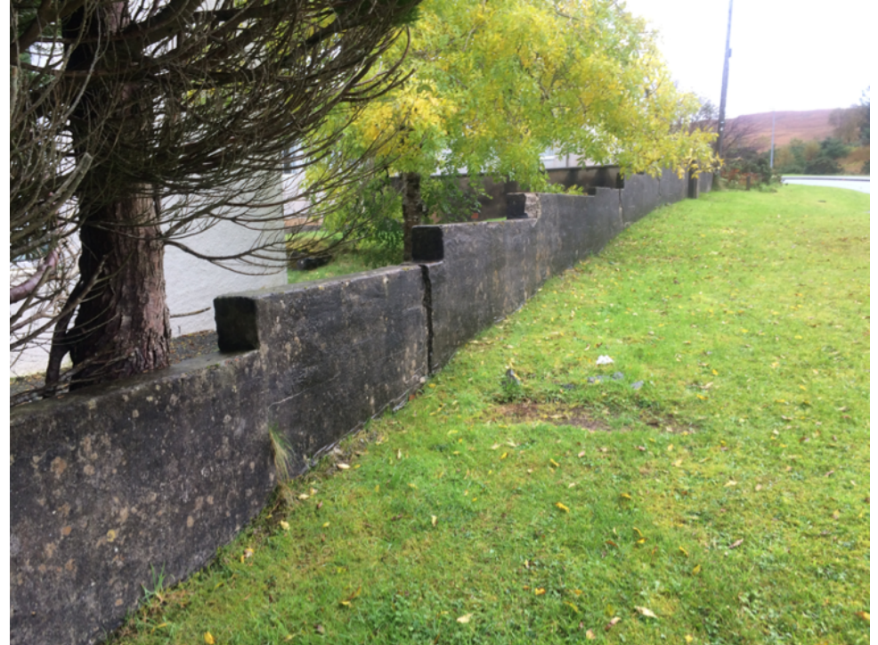
Cracks to boundary wall at west end
