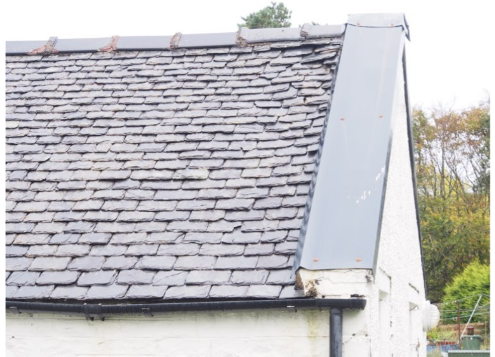
Loose slates and damaged ridge tiles on South wing
