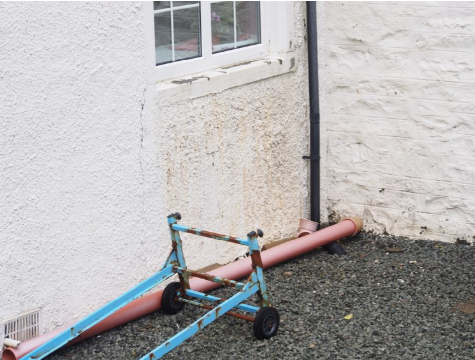
Cracked and defective render below window at south elevation
